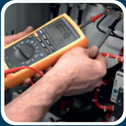
Electrical Testing Compliance and risk mitigation
